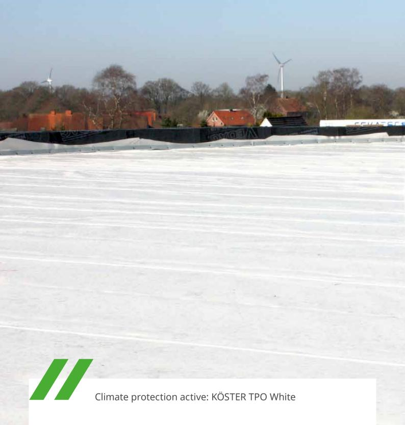
The KÖSTER TPO White is a highly reflective thermoplastic waterproofing membrane. It reflects most of the sunlight directly back and therefore hardly heats up. The roof remains pleasantly cool and air conditioning costs are reduced. That saves energy. Even further: reflected solar energy reduces global warming.
