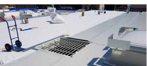
Roof waterproofing with self-adhesive TPO roofing membrane, new construction, Schwetzingen, Germany
